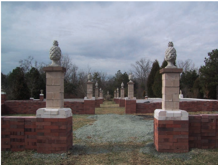
The Walled Garden under Construction
